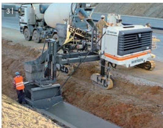
2 | Production of a reinforced concrete median barrier.
