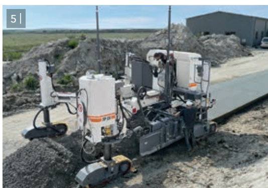
4 | Paving tracks for an agricultural road.
